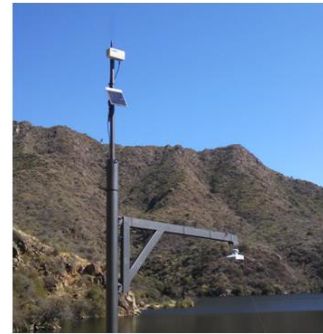
Dam water level monitoring
